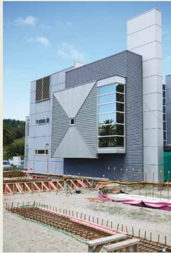
Existing elevation to be demolished
